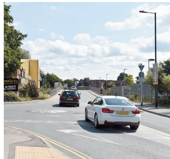
The mini roundabout by the Stafferton Link Road is due to be repositioned. Ref:133718-6
