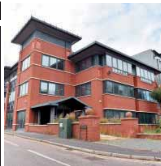
Thames House, in Marlow Road. Ref:133689-5
