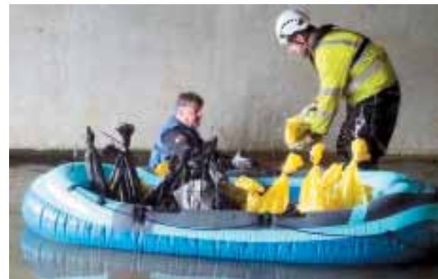
Work on the Waterways weir.
